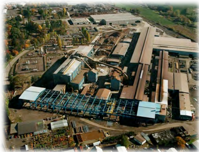
Cascade Steel Rolling Mills, McMinnville, Oregon
