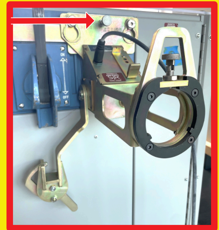
SDB MOUNTED TO CUBICLE USING CUBICLE KIT SHOULDER NUTS, SECURED WITH LOCKING PIN
