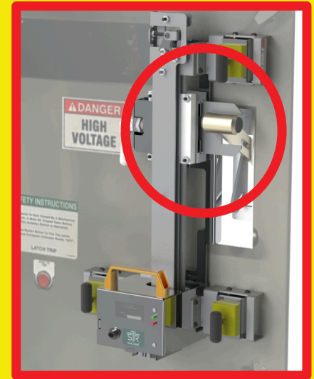
CARRIAGE ARMS CORRECTLY POSITIONED AROUND CONTACTOR OPEN/CLOSE LEVER
