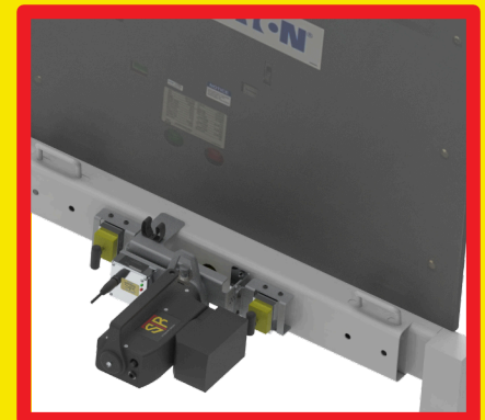
MDU WITH ATTACHED TAA PROPERLY ENGAGED WITH DRIVE RINGS AND LOCKING PIN, READY FOR SDB AND HHC COMMUNICATION CORDS
