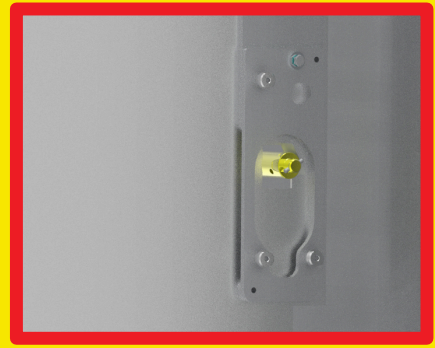
ITA ENGAGED WITH RACKING SHAFT
