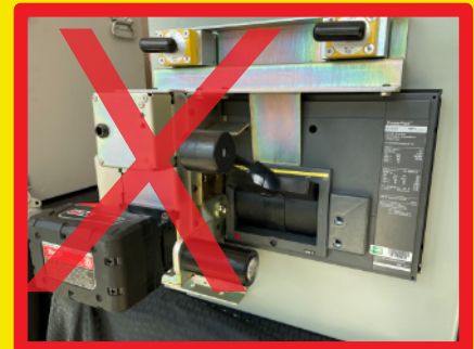
INCORRECT POSITION OF ROC HANDLE BEFORE MANIPULATING ARM ADJUSTS TO CORRECT PLACEMENT TO PERFORM OPEN/CLOSE FUNCTION
