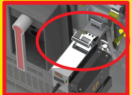
FORWARD ASSIST SPRING ASSEMBLY SECURING SDB IN PLACE AGAINST CUBICLE
