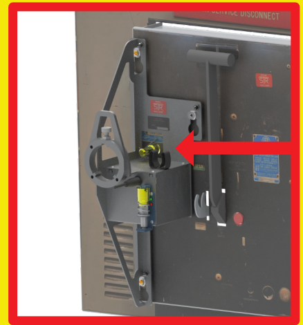
SDB SUSPENDED FROM SHOULDER BOLTS; ITA INSERTED INTO RACKING PORT
